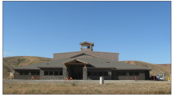
The new Operations & Maintenance Building for Phase I of the Lower Snake River Wind Project includes offices, warehouse space and a workshop for the 25 permanent employees of PSE and Siemens Energy who are based there.
