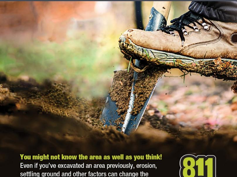
settling ground and other factors can change the depth and location of utilities over time. ALWAYS contact 811 before putting your shovel to the ground!
