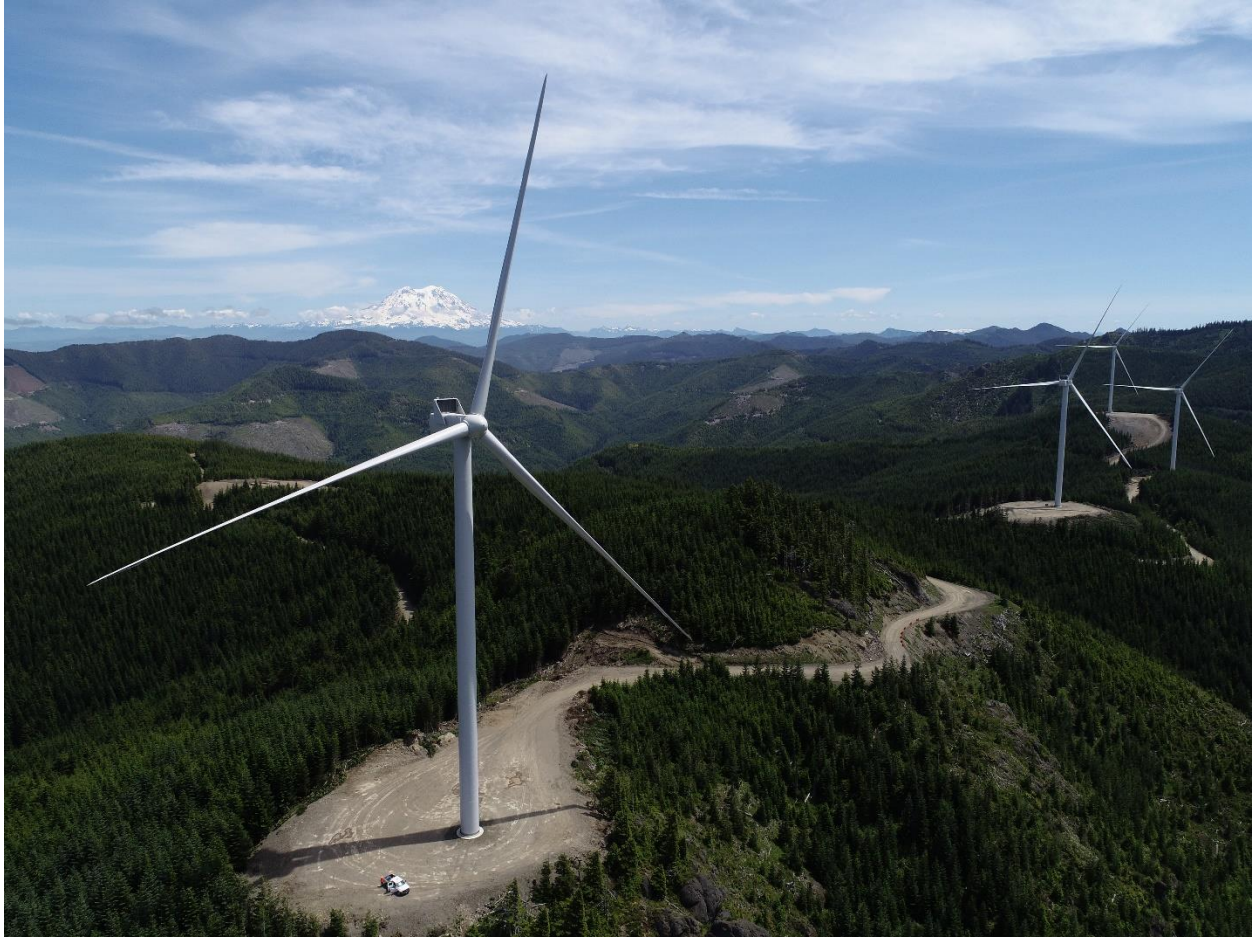
Skookumchuck Wind Facility, Southern Power
